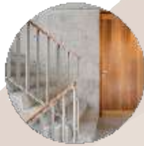
IRON GUARD RAIL
